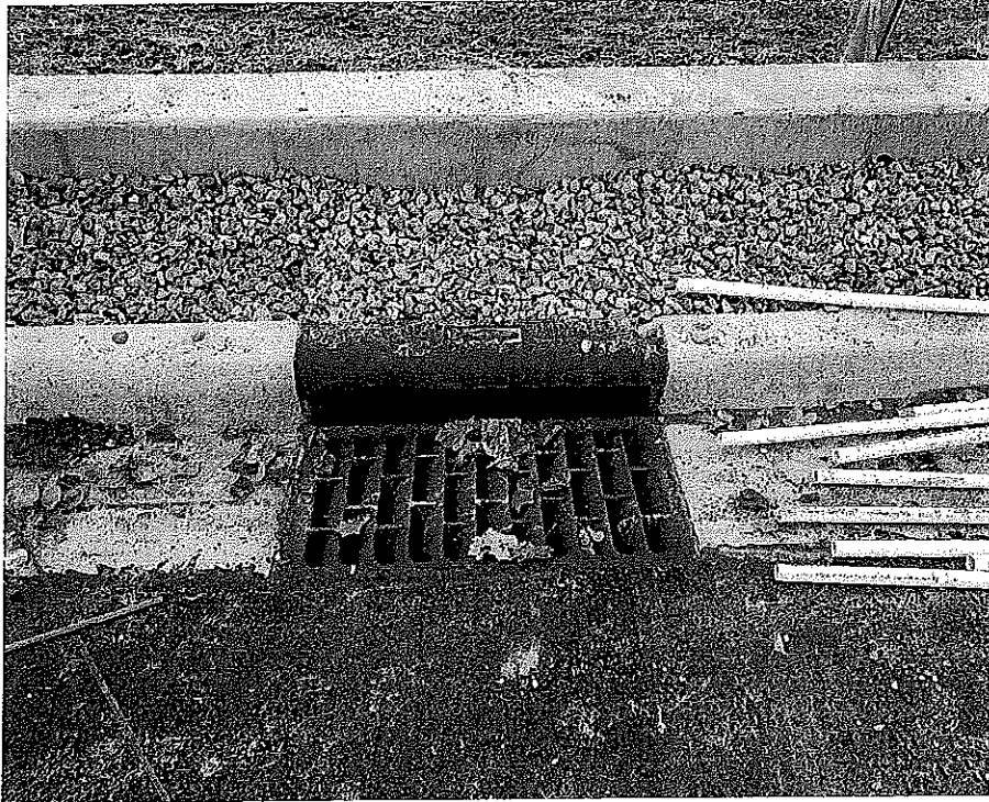
Outside of Catch Basin – CB 8
