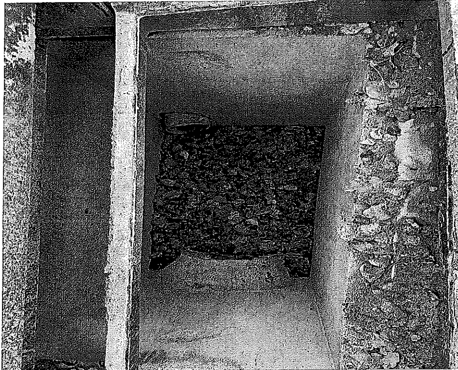
Inside of Catch Basin – CB 7
