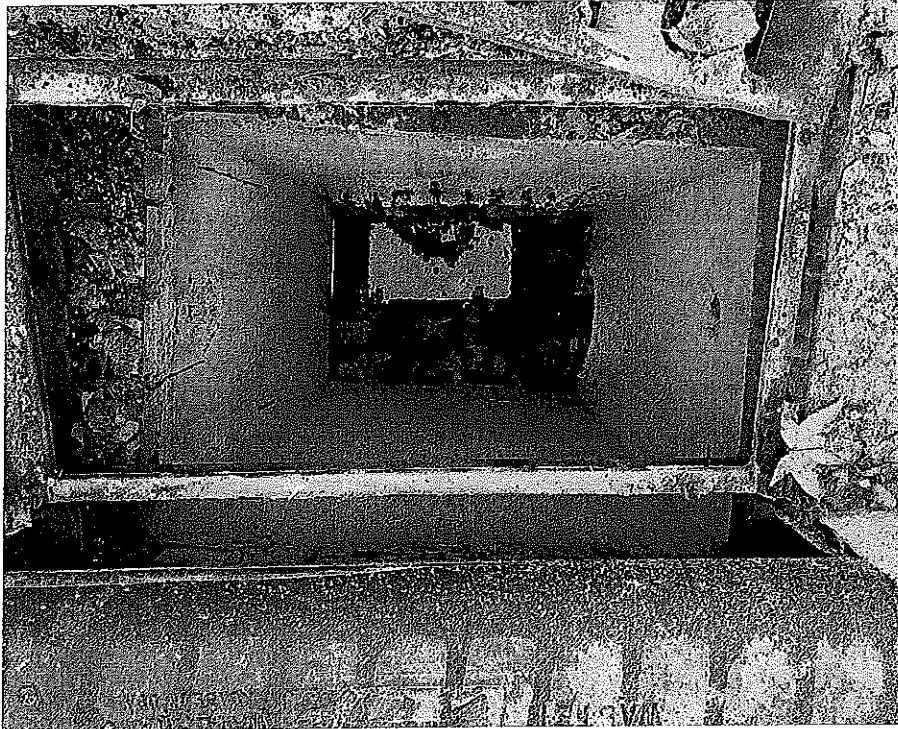
Inside of Catch Basin – CB 6
