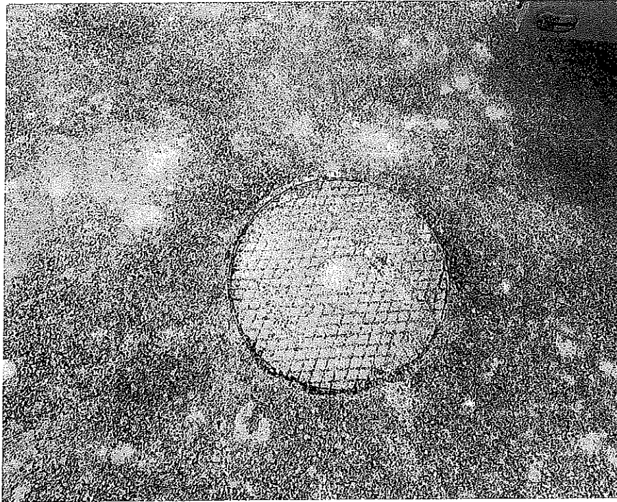
Outside of Storm Manhole – MH 10
