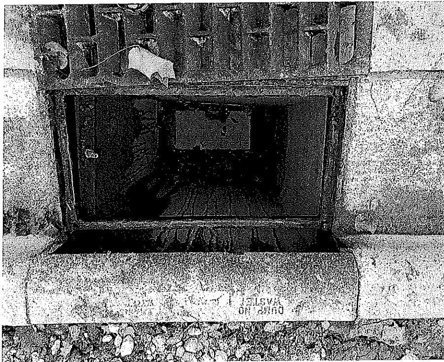
Inside of Catch Basin – CB 2
