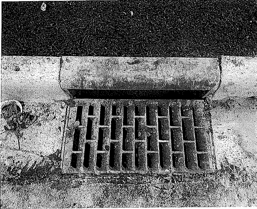
Outside of Catch Basin – CB 9
