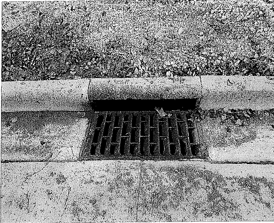
Outside of Catch Basin – CB 2
