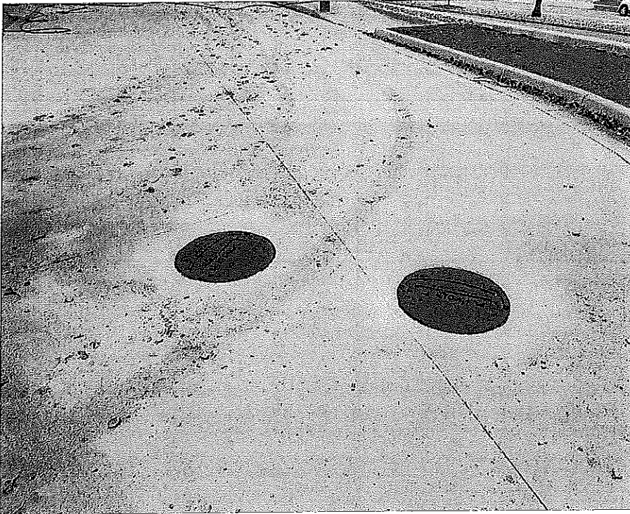
Outside of Outlet Structure – OS 1
