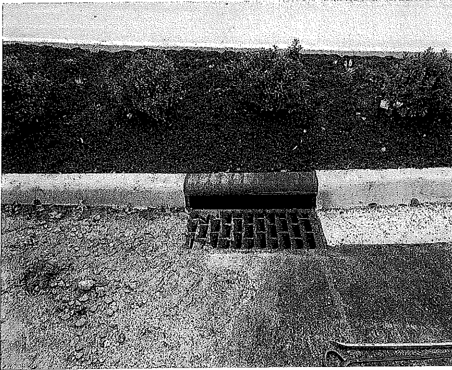
Outside of Catch Basin – CB 6
