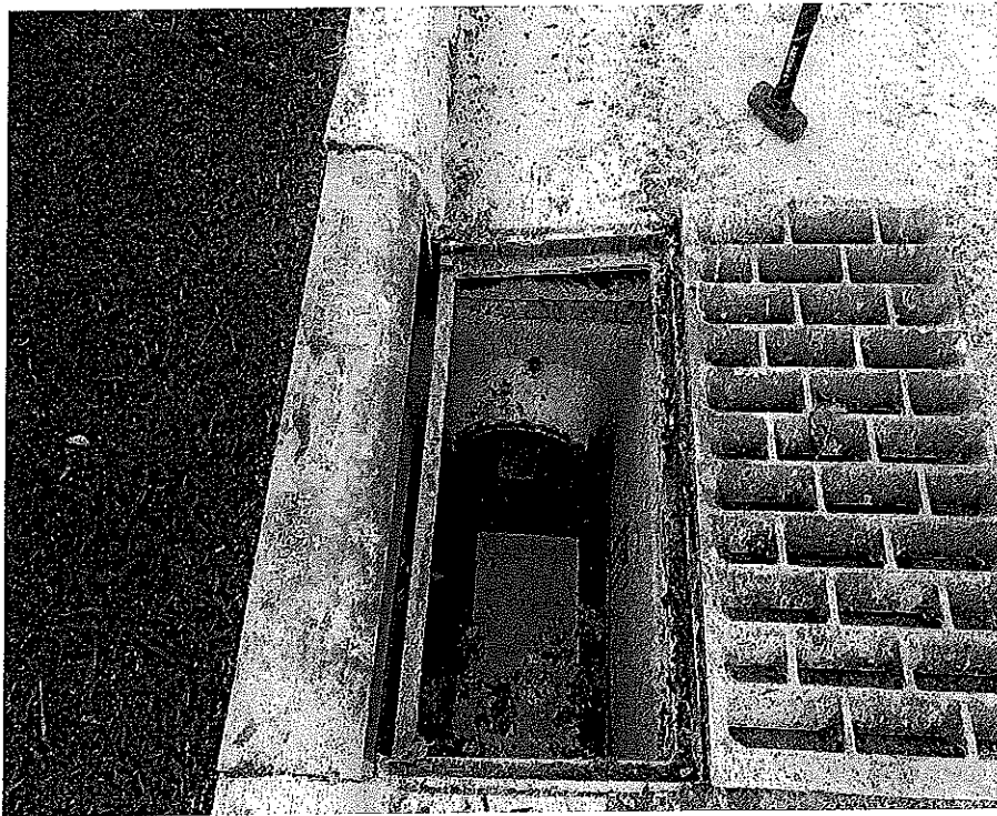
Inside of Catch Basin – CB 9
