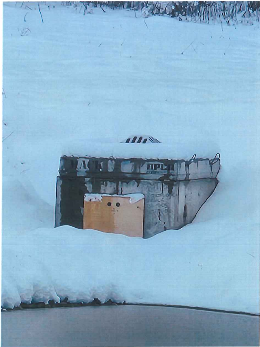
Pond Outlet Structure
