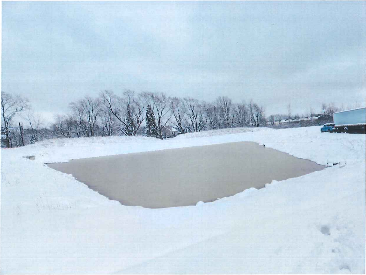
Storm Water Management Pond
