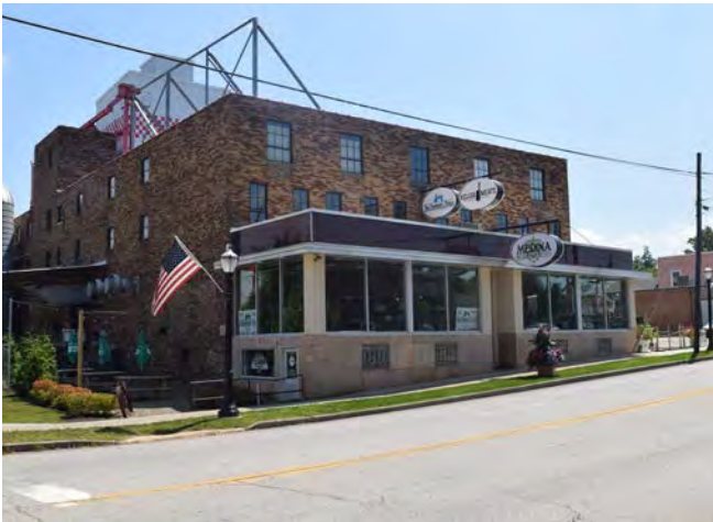
View of the redeveloped Farmer's Exchange building on South Court Street.
