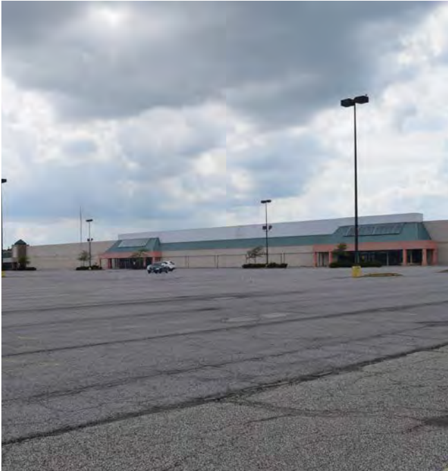
Former Kmart building and parking lot.
