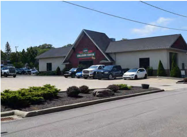
Auto Collision Center located at the intersection of South Court Street and Mill Street.
