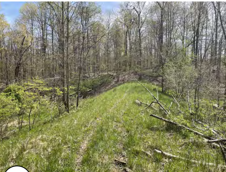
5 Use Levee: Existing levee could route trail over creek
