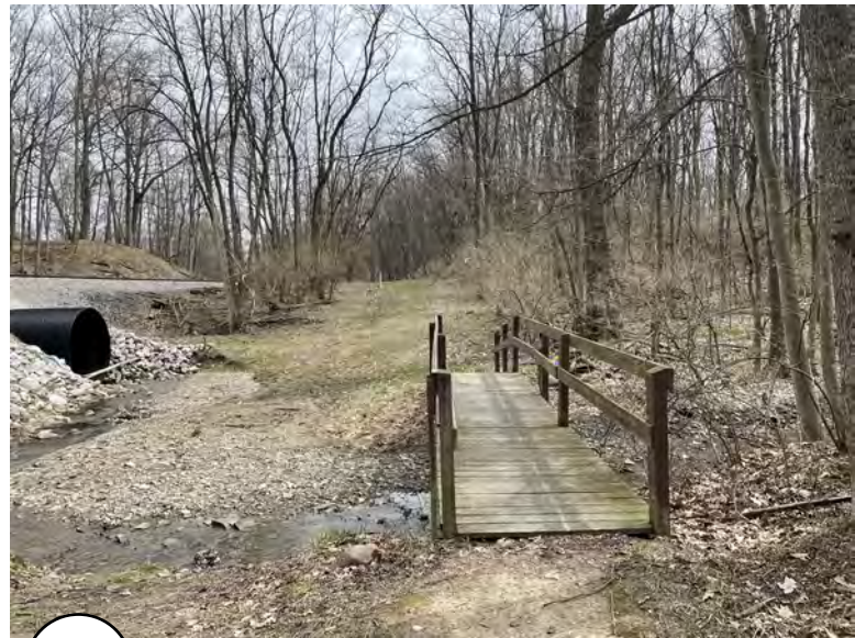
2 Run along sewer line: Sewer line runs parallel to rail line, path cleared ~1,200 Ft
