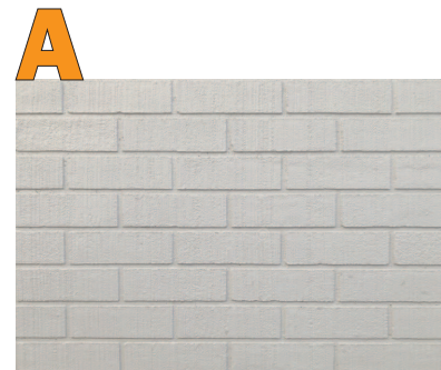
A MATERIAL: MODULAR BRICK PATTERN: RUNNING BOND FINISH: PAINTED SW 7015 REPOSE GRAY
