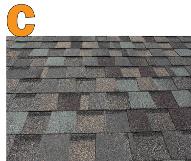
MATERIAL: DIMENSIONAL SHINGLE PATTERN: STANDARD FINISH: TBD
