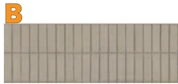
MATERIAL: MODULAR BRICK PATTERN: SOLDIER COURSE (VARIES) FINISH: PAINTED SW 7017 DORIAN GRAY
