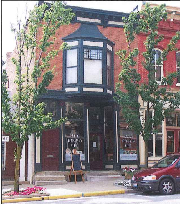
Trees, plantings, and signage contribute to the streetscape.
