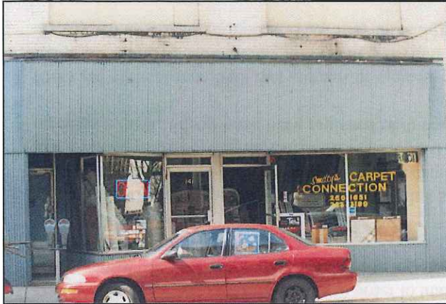
Storefront had been altered from its original appearance.
