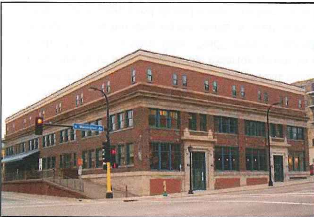
Example of a poorly designed roof addition to an existing structure
