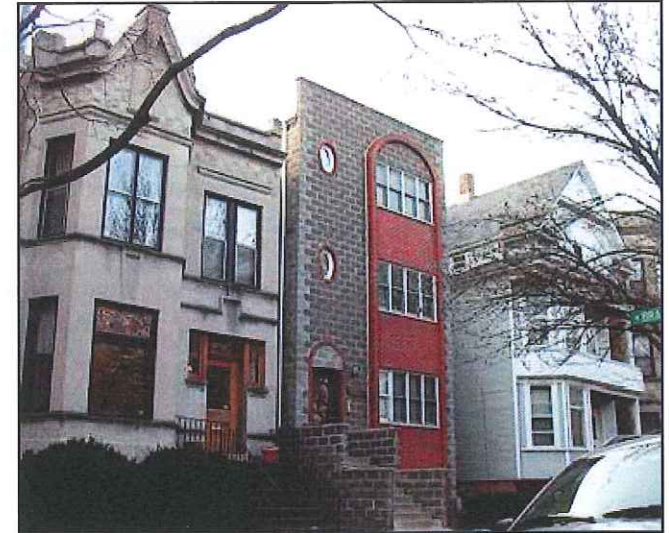
Example of an infill that poorly relates to adjacent existing structures
