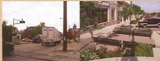
Infrastructure to support development
