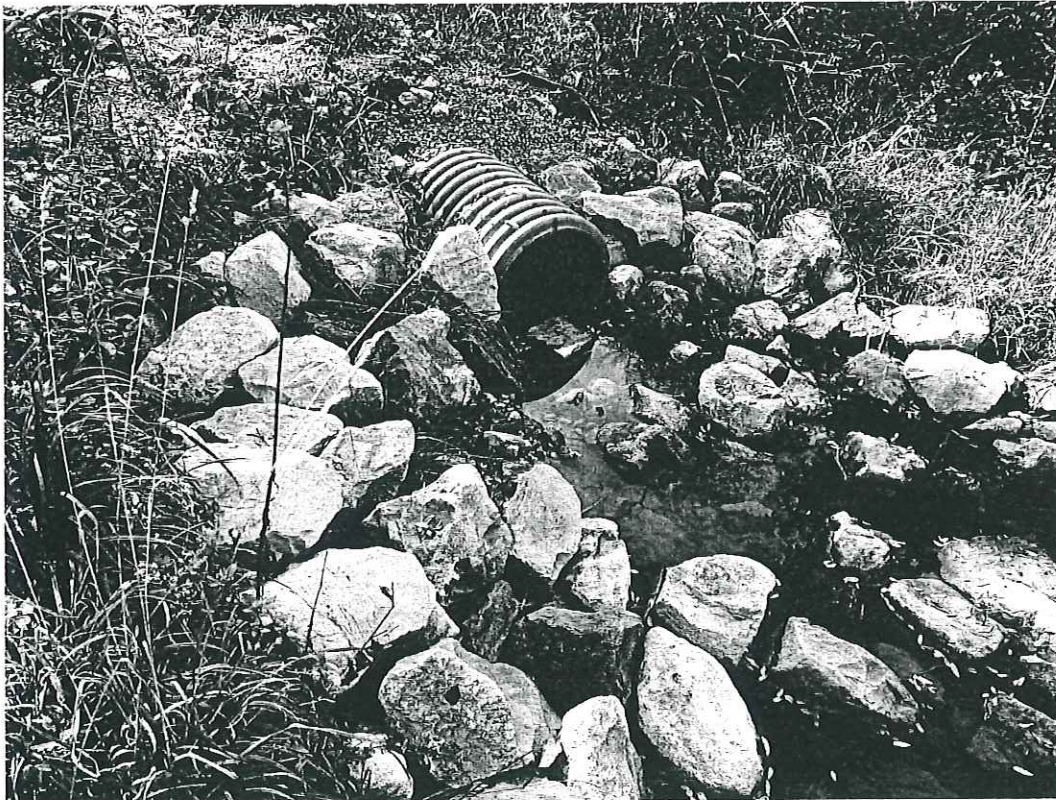
OUTLET STRUCTURE TO SWALE
