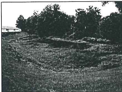
Well maintained dry detention basin. Forebay in the background. Main pool area receives periodic mowing to maintain vegetation. Credit: Cuyahoga Soil & Water Conservation District
