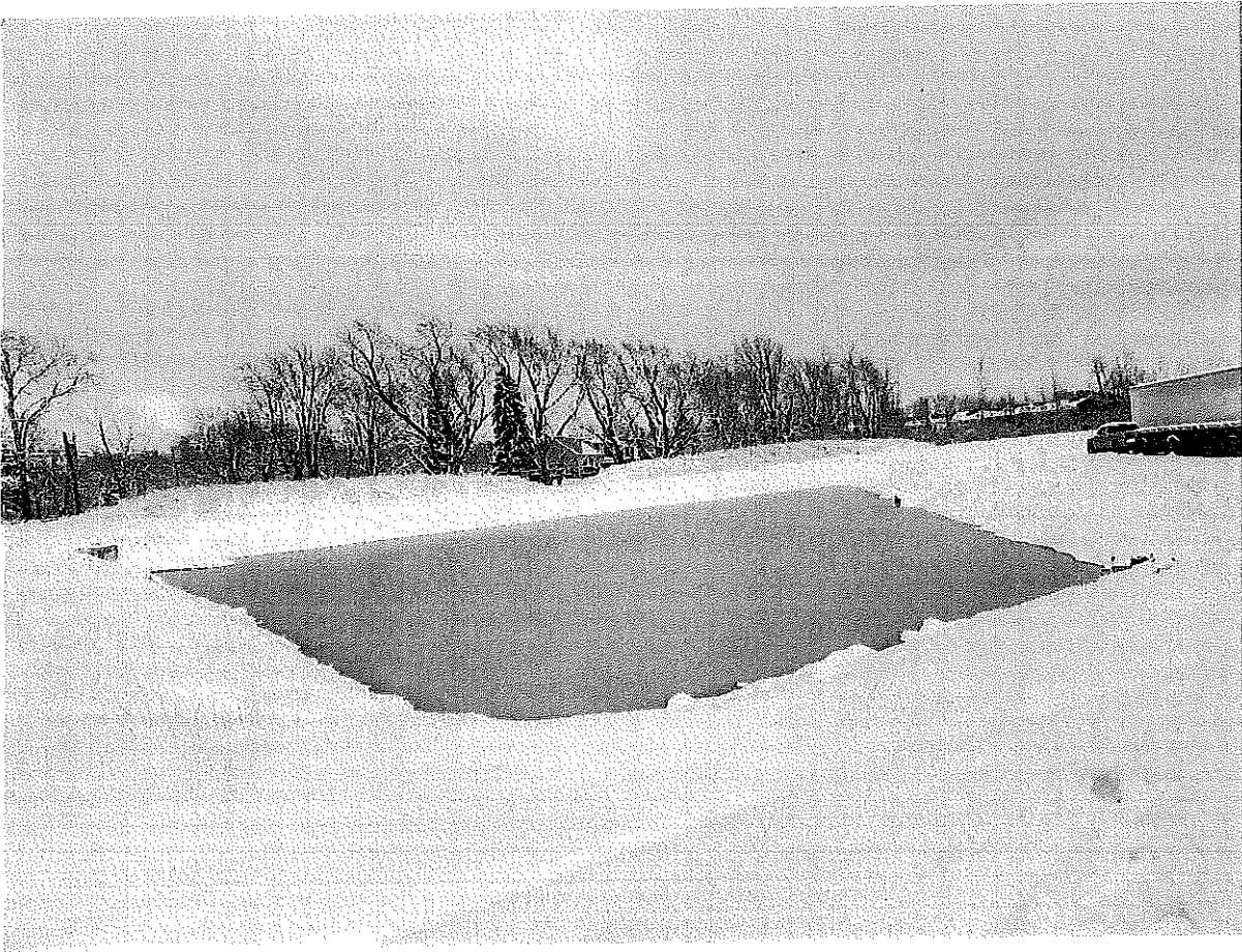
Storm Water Management Pond
