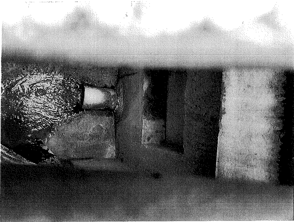
Inside of Outlet Structure
