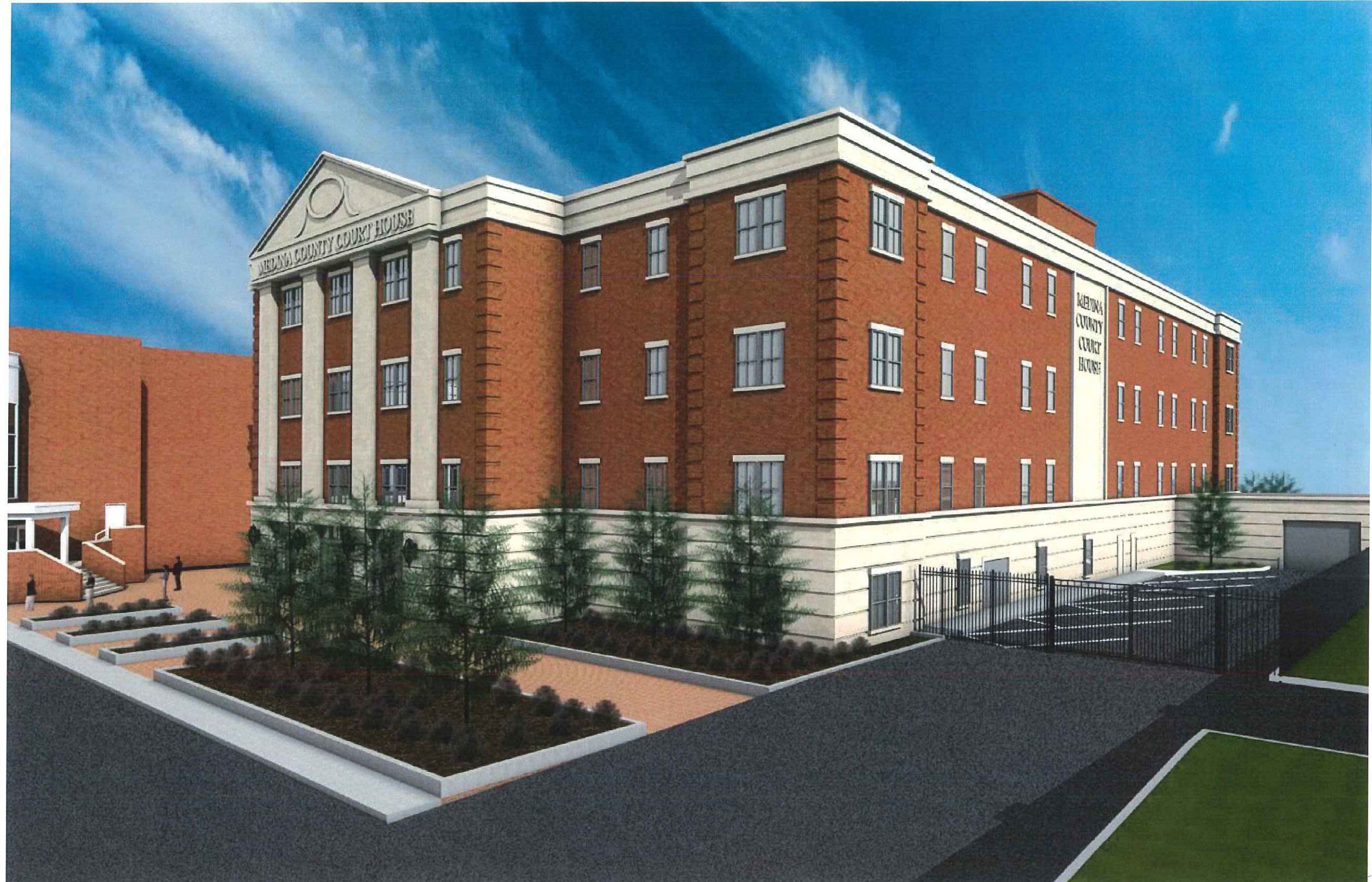
VIEW LOOKING NORTHWEST FROM S. WASHINGTON STREET
