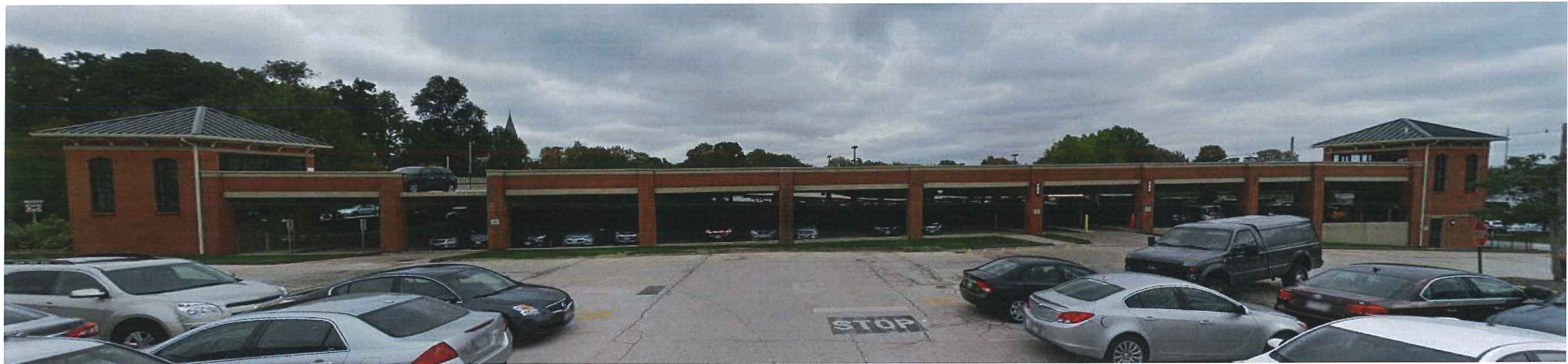
Parking Garage - West Side
