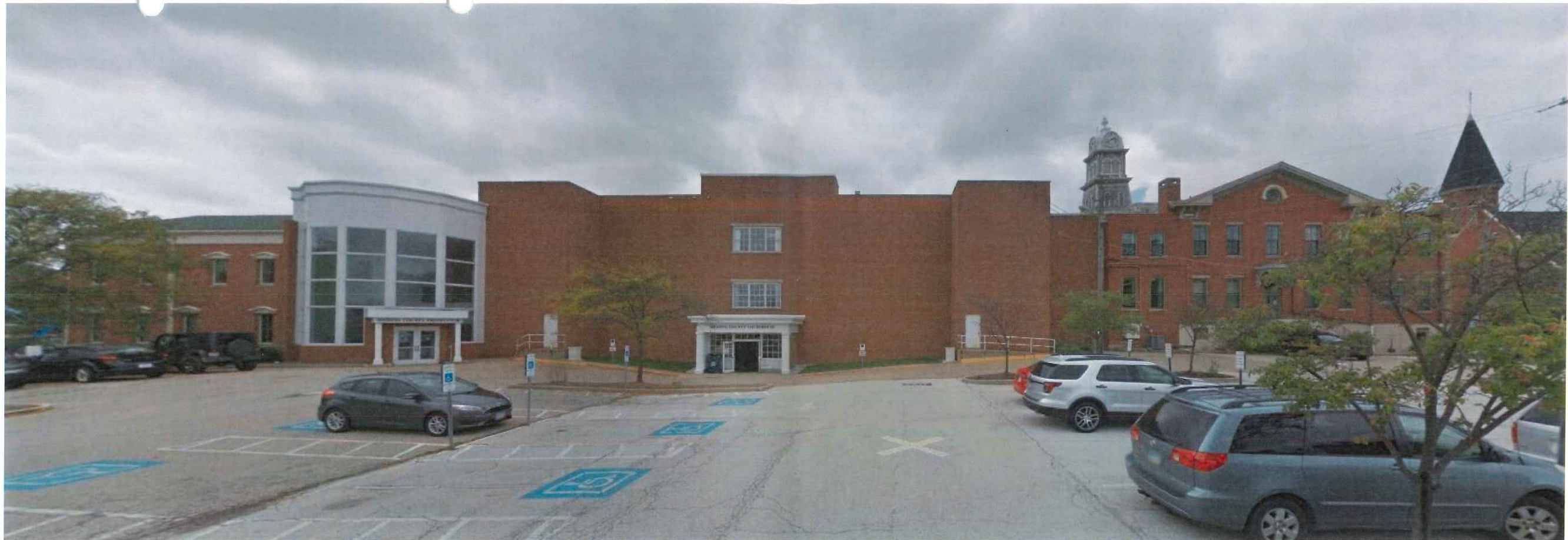
Courthouse Block - East Side
