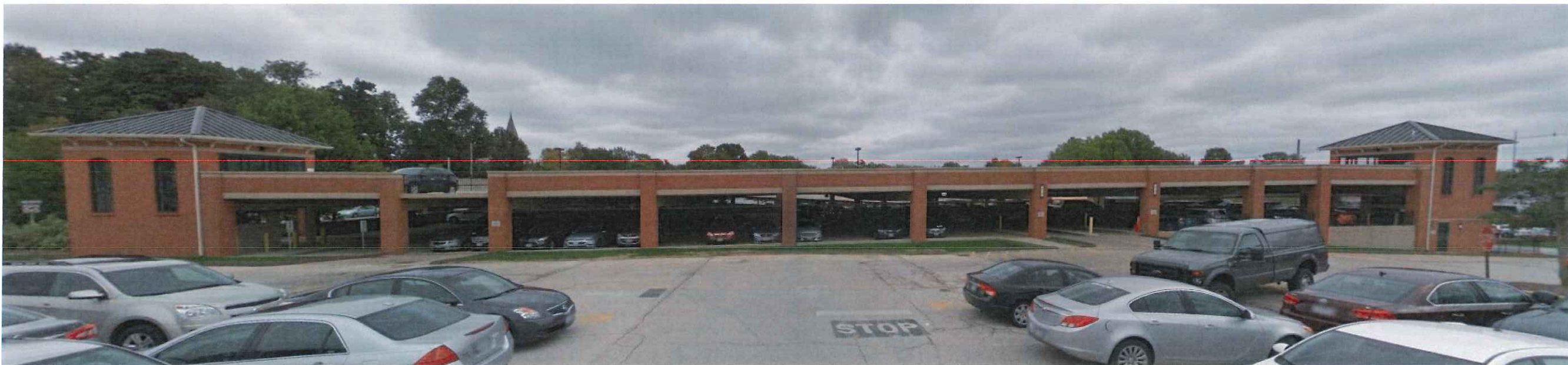
Parking Garage - West Side
