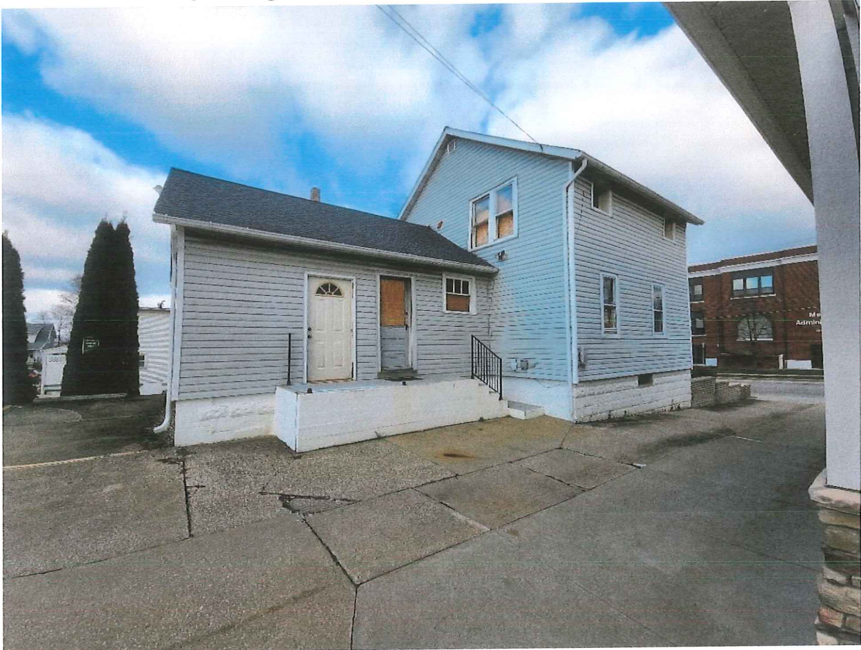
South Elevation, facing north
