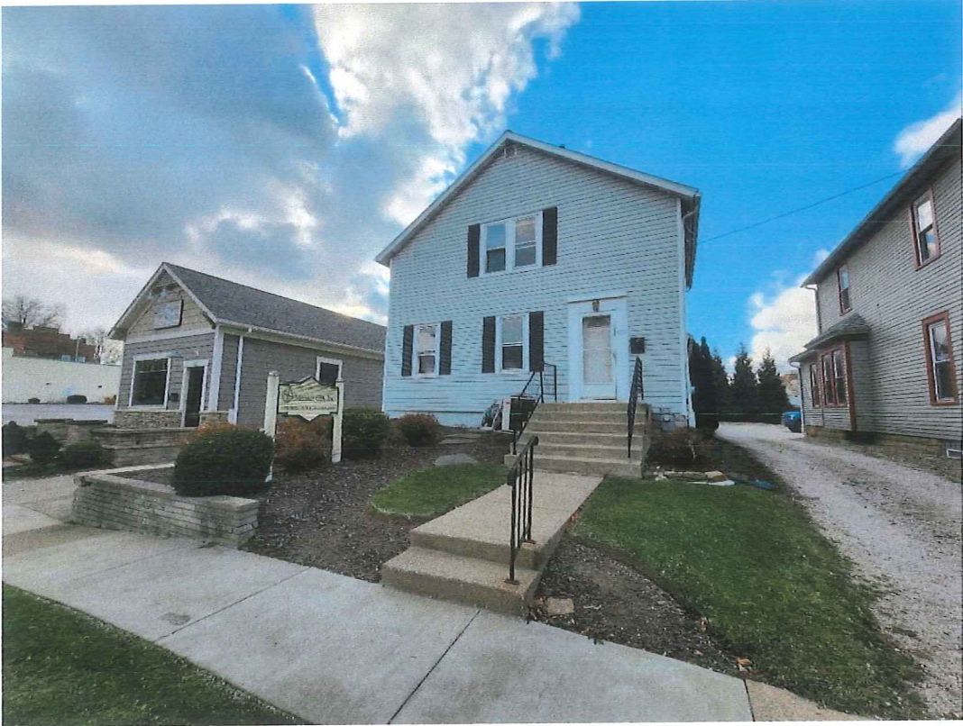
East side (North Broadway) looking west (Streetside)
