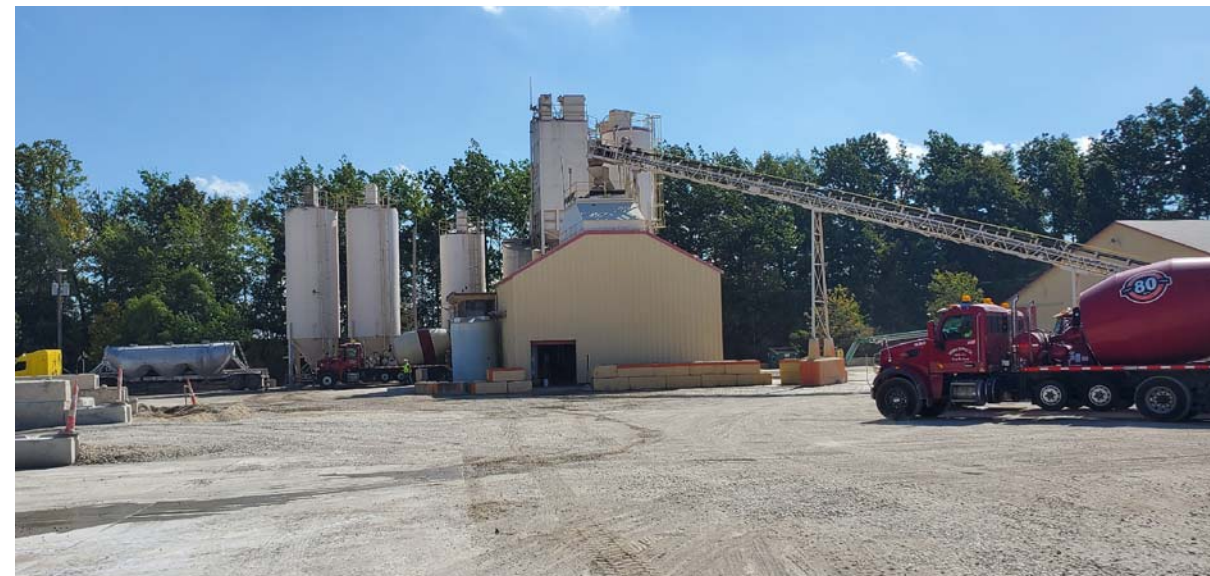
1 REFERENCE IMAGE SD-1 EXISTING BATCH PLANT TO BE REMOVED
