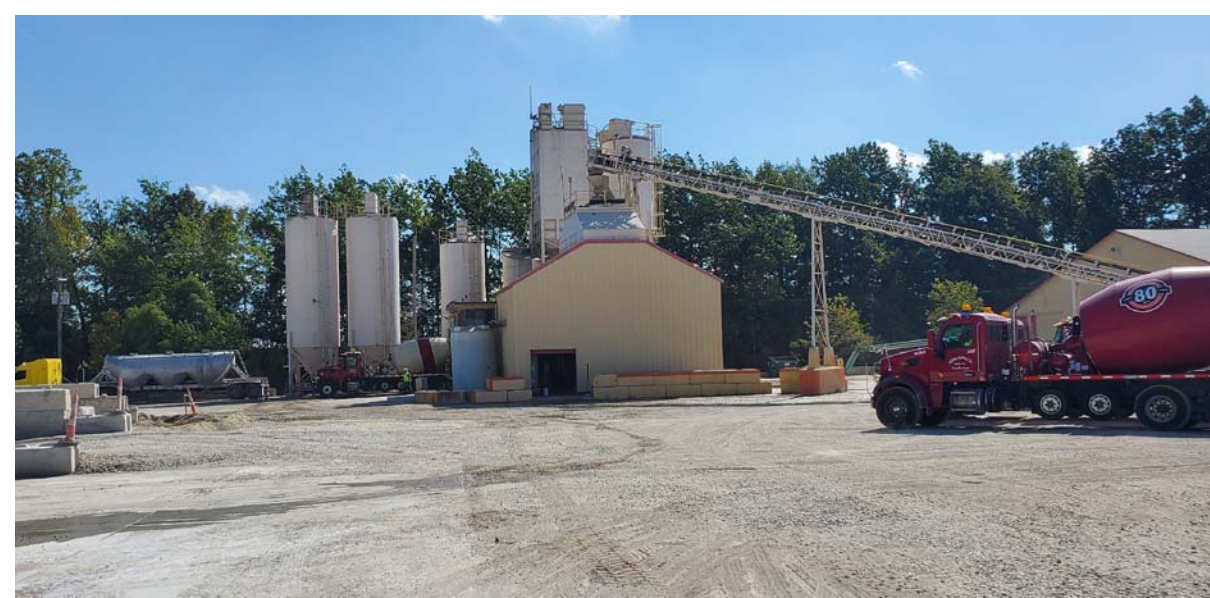
1 REFERENCE IMAGE SD-1 EXISTING BATCH PLANT TO BE REMOVED
