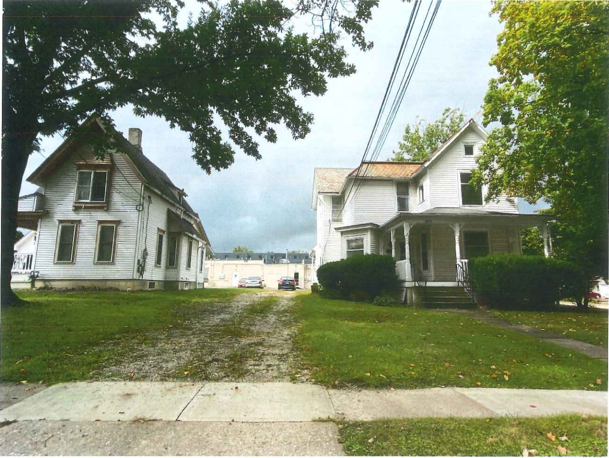
Front view of N. Broadway homes
