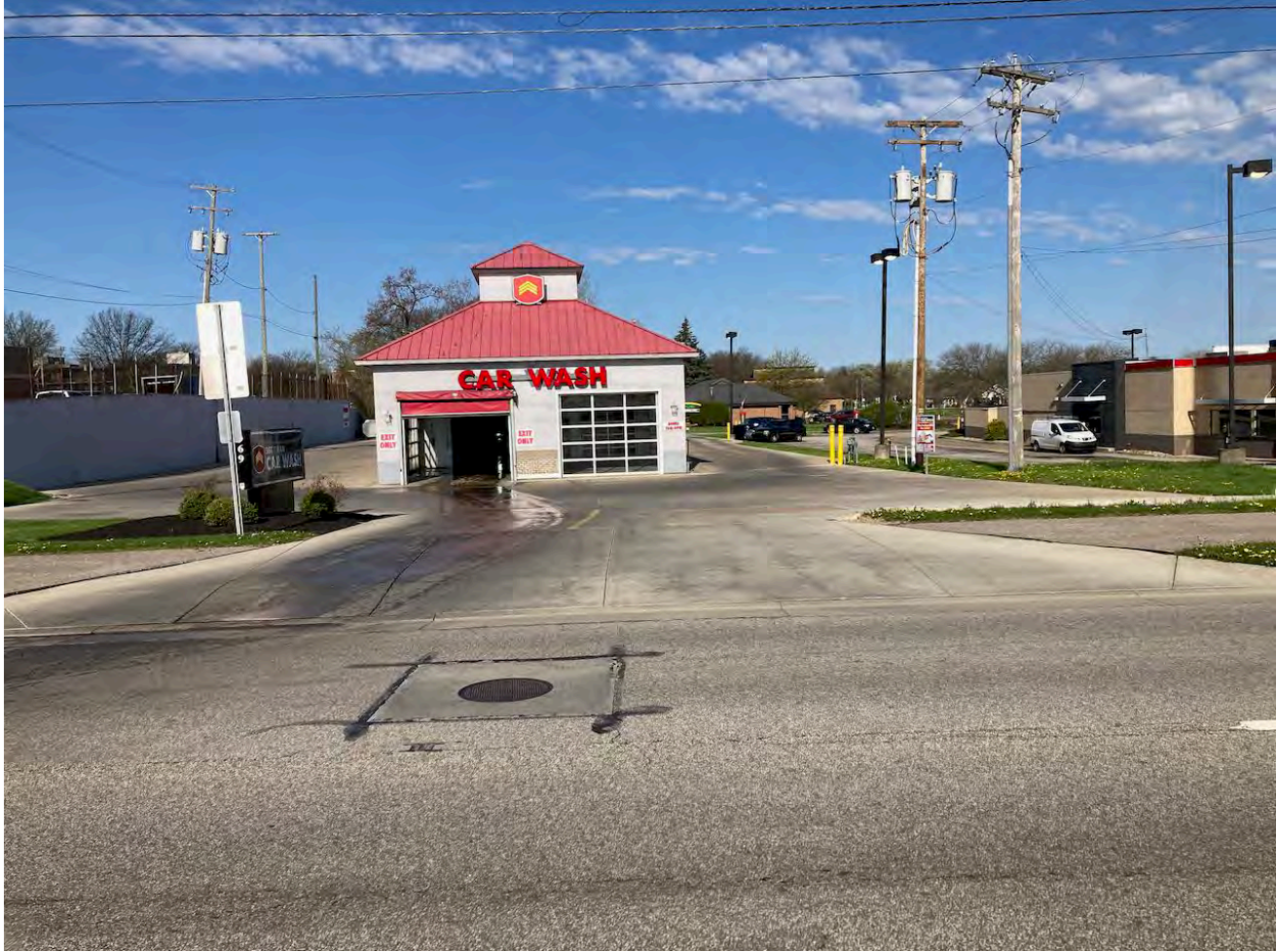
North Court Street-Front view
