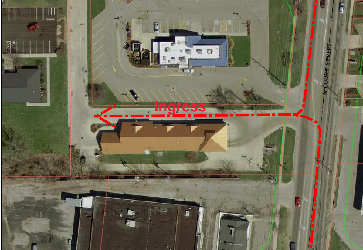
Prior to North Court Street Reconstruction
