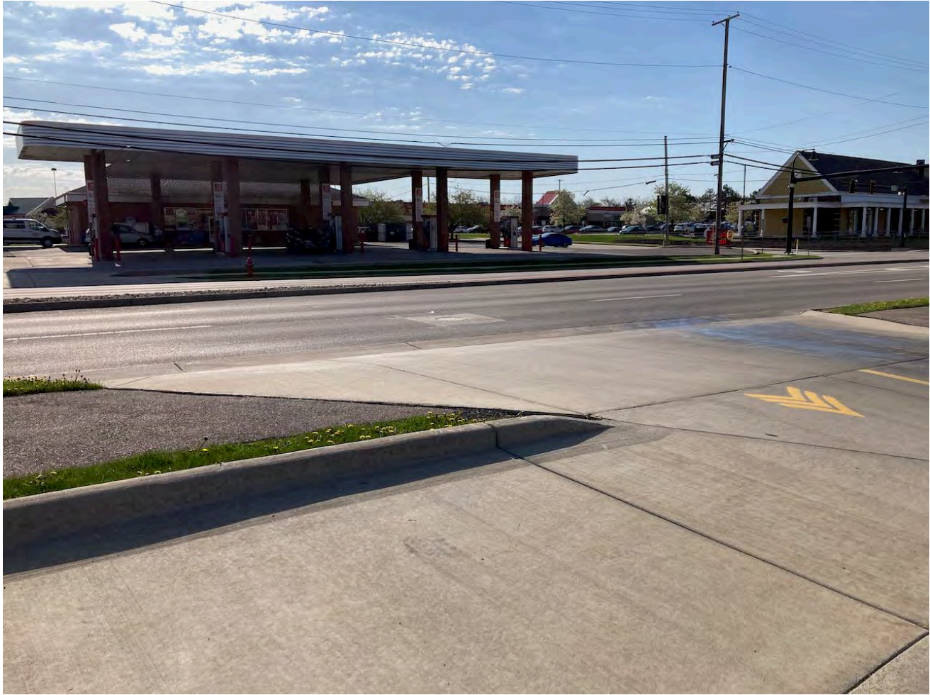
North Court Street-entry-north side
