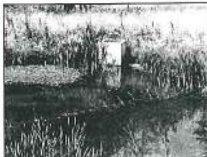
Outlet structure with multiple drains free of obstruction such as vegetation, trash or sediment. Credit: Summit Soil & Water Conservation District
