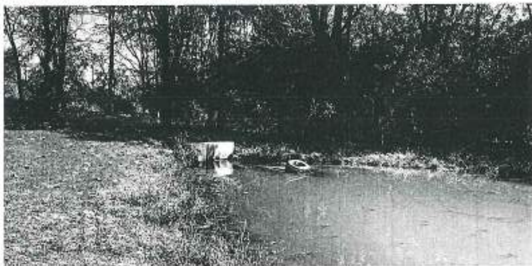
OUTLET STRUCTURE TO SWALE
