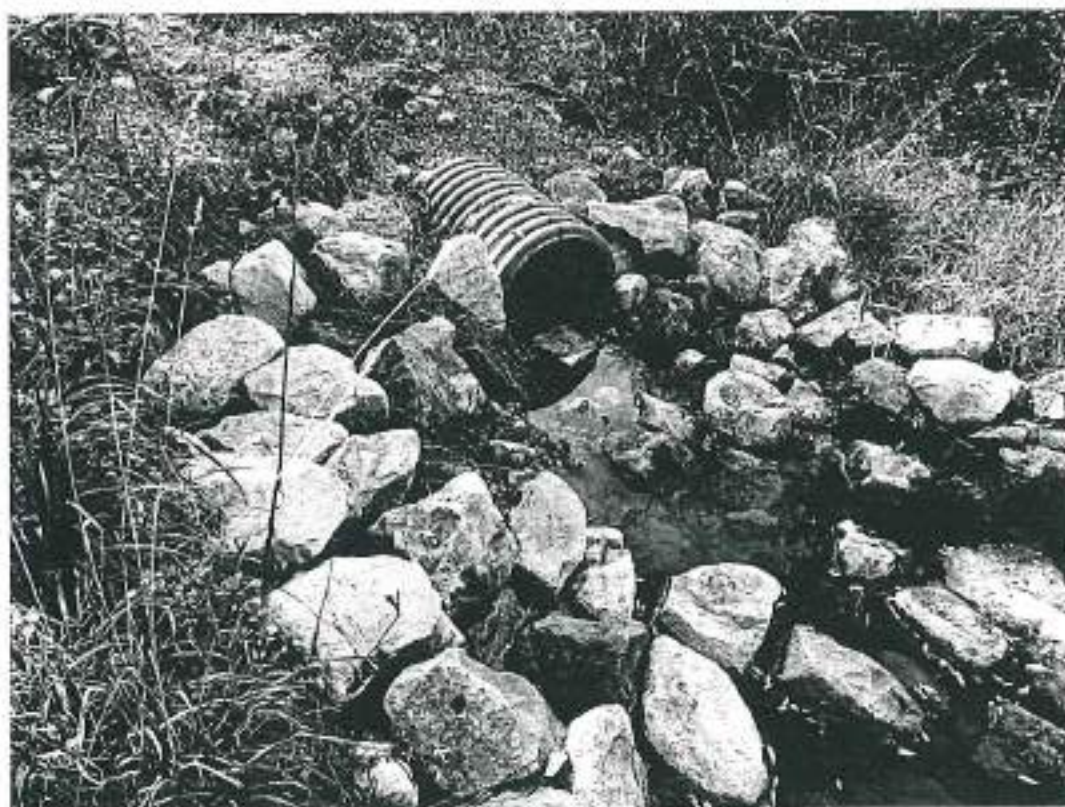
OUTLET STRUCTURE TO SWALE
