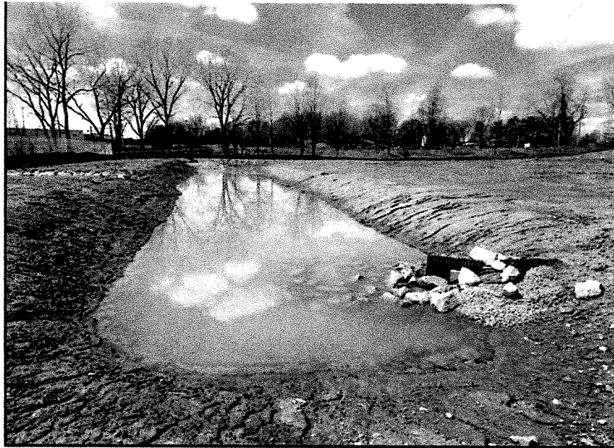
JPA Trucking – Sediment/Dry WQ Detention Basin Inlet View
