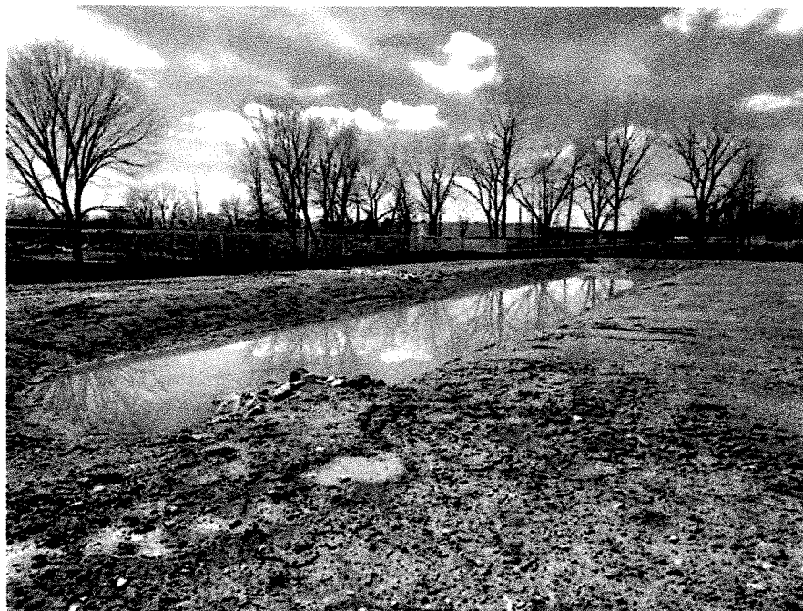
JPA Trucking – Sediment/Dry WQ Detention Basin Overall View
